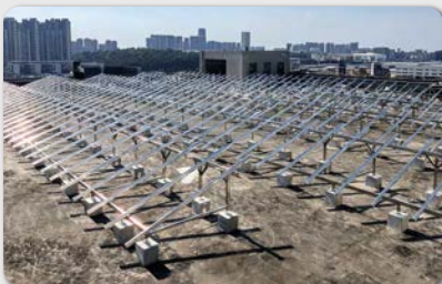
Column fixation, mounting installation
