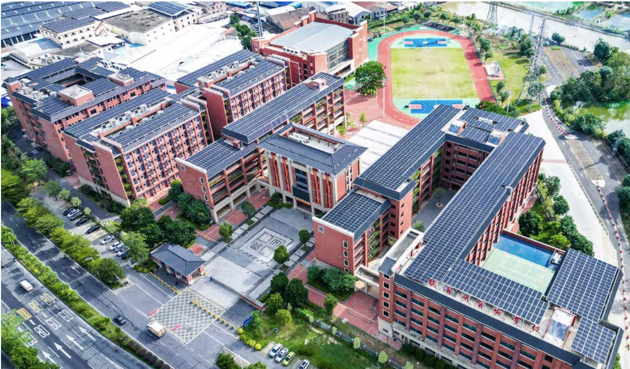
📍 Tingyin Lake School(Foshan) | Installed Capacity: 1.4MW | 1st-Year Generation: 1.6GWh
