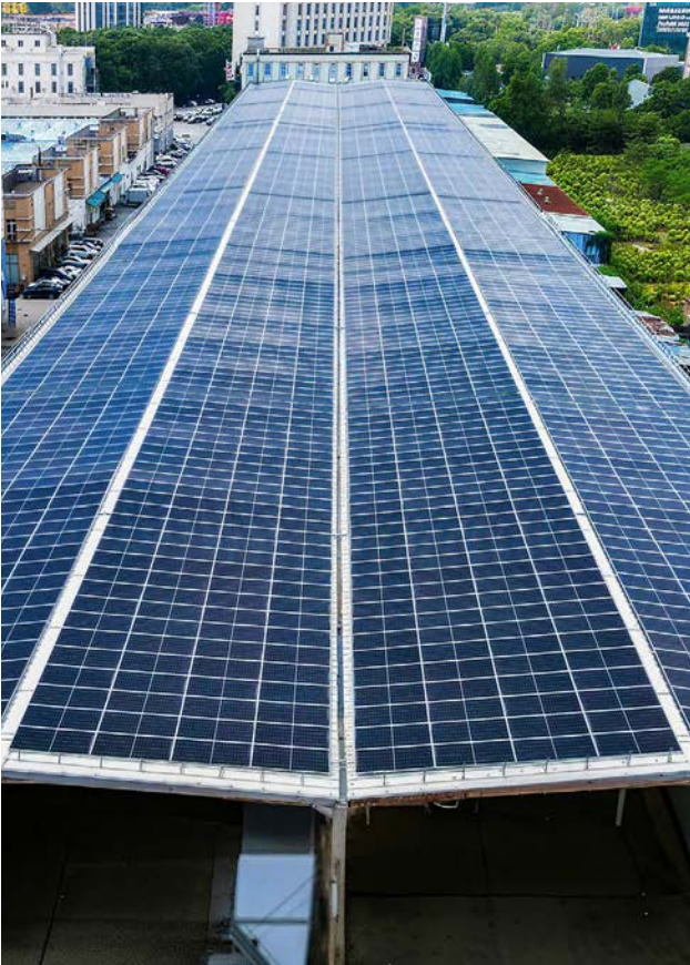
📍 Guangfo Auto City(Foshan ) | Installed Capacity: 8.75MW | 1st-Year Generation: 9.65GWh
