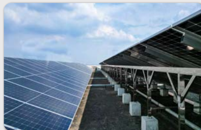
Installation of PV panels
